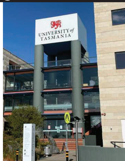
The award-winning Centenary Building. UTAS wants to demolish it, moving the Business School to the controversial Melville St building.
